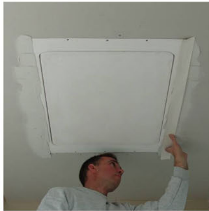
2. Apply drywall tape, also covering seams and screws.
