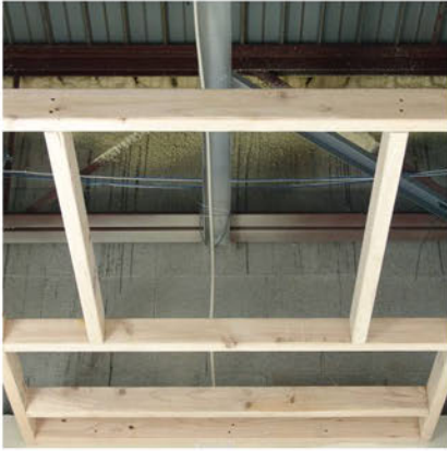
1. Frame out location of the panel.
